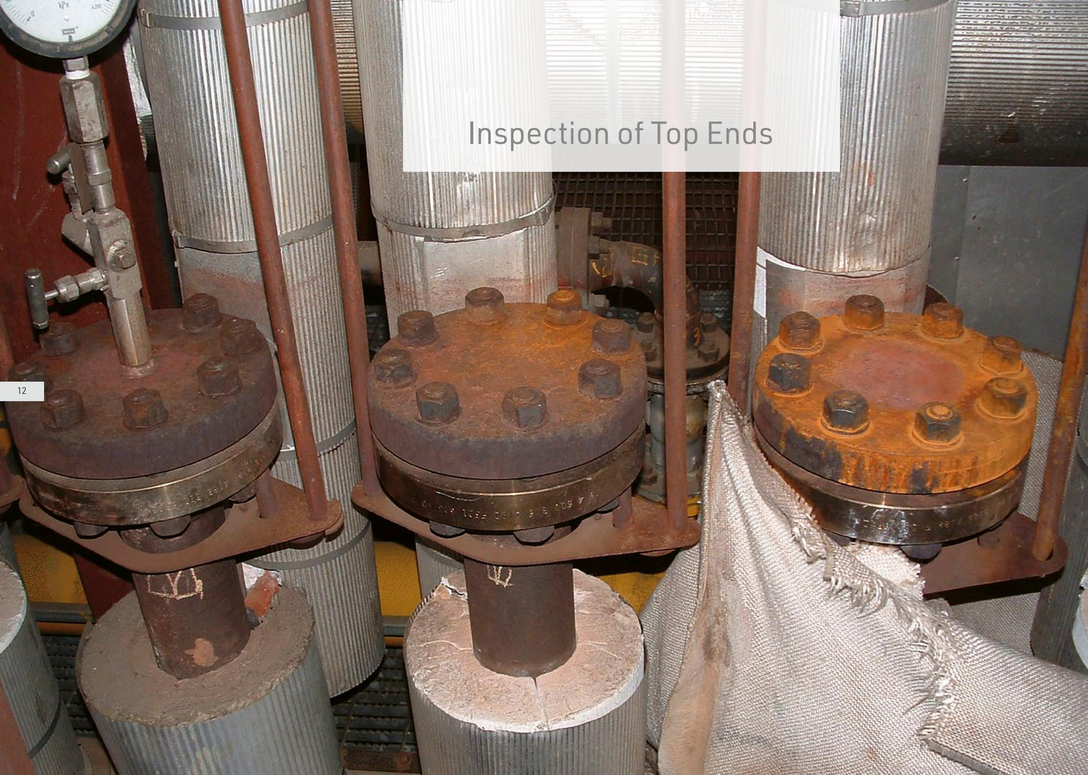
The historically accepted standard for examining in-service reformer tubes in steam methane reformers (SMRs) has been to inspect the heated length of the tube within the furnace. However, recent trends have changed that perspective, due to the discovery of internal defects and damage in these heretofore uninspected portions of the tube at the top ends in some plant designs.
